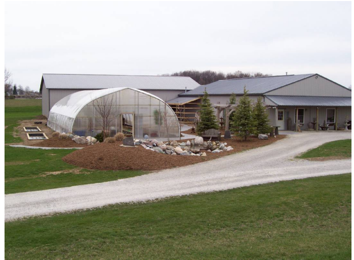
Expansion project at Woodland
